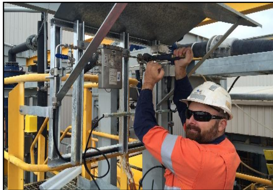
Instrowest technician commissioning the new Hanbay actuator and Siemens Coriolis flowmeter
